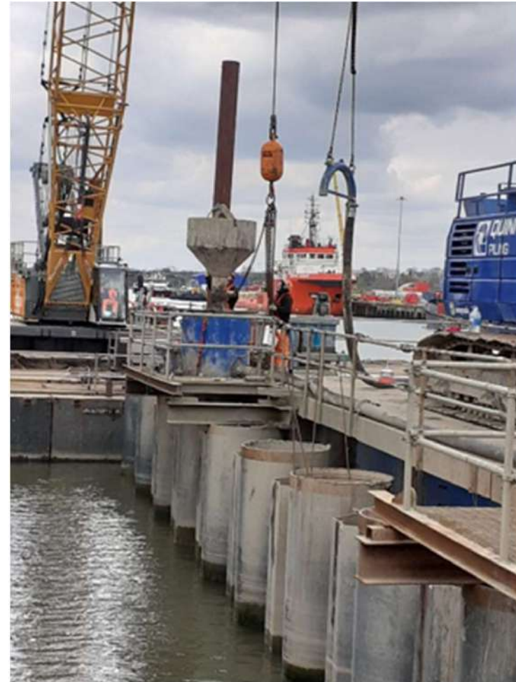
Pier 4 Rotary Bored Piling: Concreting Operation
