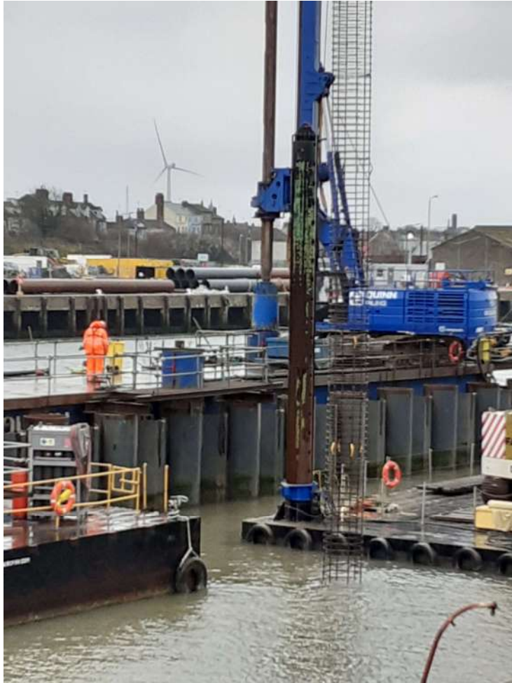
Pier 4 Rotary Bored Piling: Cage Installation
