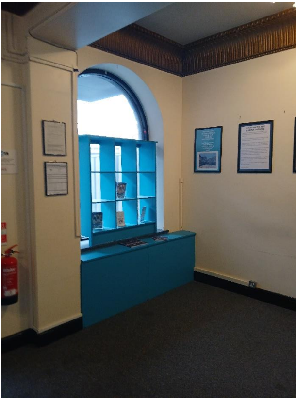
Foyer area showing routes for CCTV and data cables.
