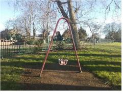
Though some of the equipment is old, it is generally in good order overall, with the main issues picked up on the last inspection being worn paintwork, surface corrosion and rust, which are all treatable. The grass mat surfacing has however become compacted and will need replacing. The site was assessed as 'low risk' overall.
