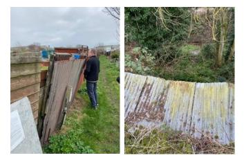
Fencing in the allotment requires to be monitored and repaired where required as some were seen to be slopping over and could possibly fall over and injury a person.
