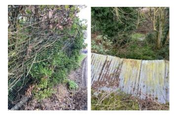
The permieter fencing was an issue in two sections, by the road the brambles were overgrowing and stretching the fencing over. This should be addressed as the issue will only get worse with time. The forth allotment areas perimeter fencing was also flat over the Gelp side. This will need to be made safe to prevent a potential fall.
