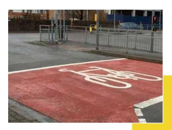
Changes to junction design to accommodate more cyclists – for example, extending Advanced Stop Lines at traffic lights to the maximum permitted depth of 7.5 metres where possible.
