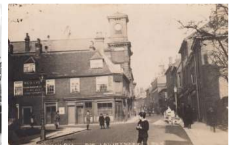
1897 photograph of the High Street showing the 1859 Town Hall Photo Credit: Alice Taylor
