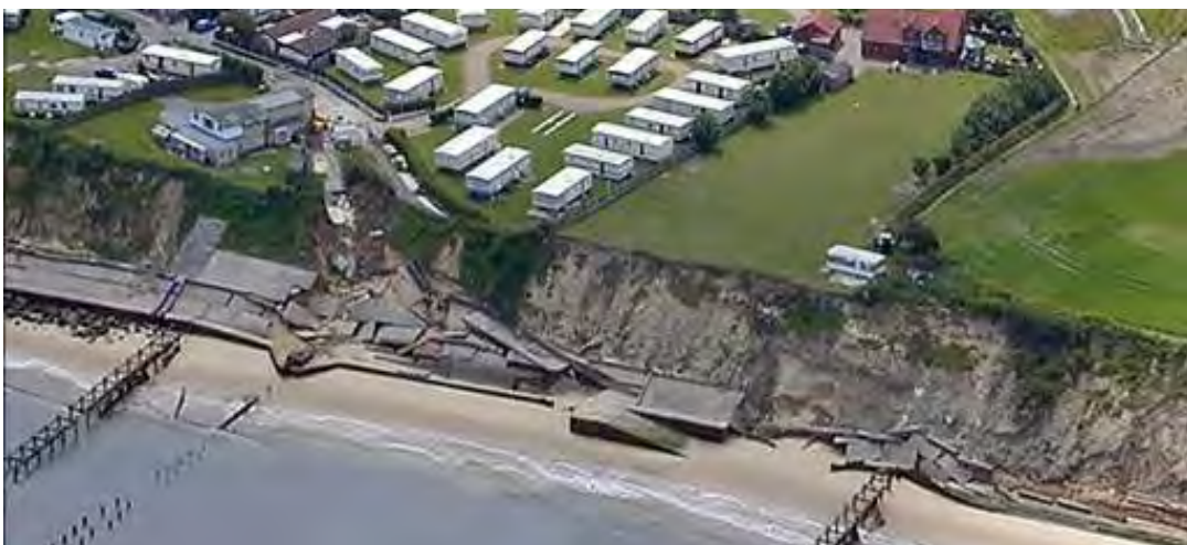
Aerial view of Corton seawall collapse
