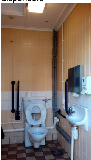
Disabled toilet, basin, lagged pipes, hand rails
