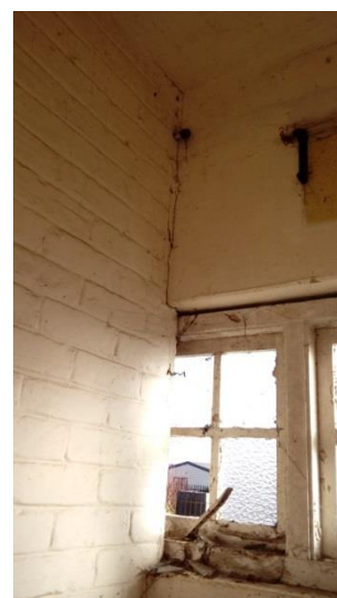
4. Capped pipe in disused toilet
