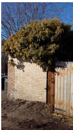
Ivy overgrown roof tiles. Note: Asbestos soffits
