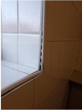
To avoid ingress of water or excessive damp, it is suggested that these openings be replaced by sealed double-glazed windows, with motion-activated lights and an extraction fan in each toilet. The condition of the locked disabled toilet is not known.
