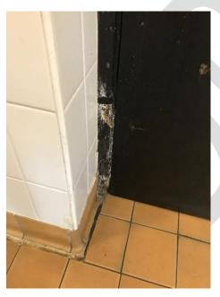
Door frame showing signs of water damage. Likely caused by continual floor mopping rather than water permeation.
