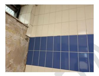
Evidence of blown plaster leading to tiles falling. .
