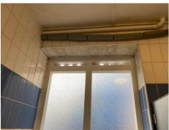
Plaster blown above window frame - tiles removed
