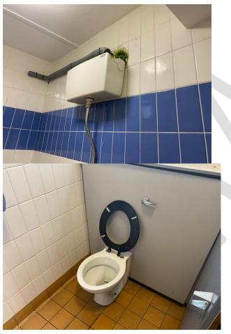
Evidence of algae spread on overhead cistern. Ball valve adjustment required and deep clean.
