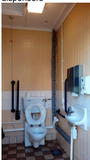
Disabled toilet, basin, lagged pipes, hand rails
