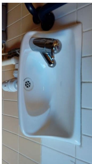
Disabled wash basin. NOTE: Thermal Mixing Valve (TMV) tap.
